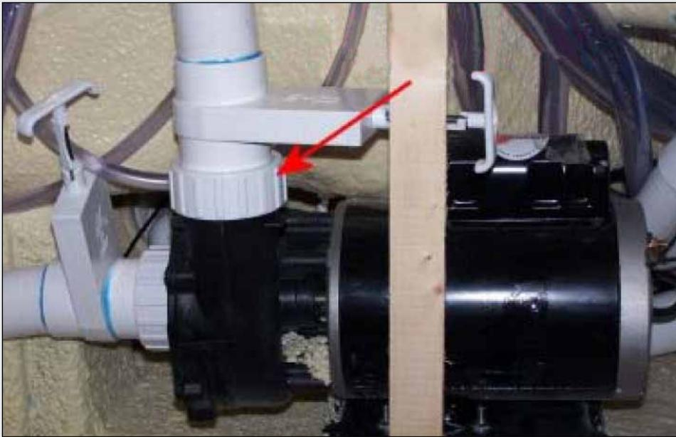
FIGURE 1.5 : HEATER UNION; LOOSEN UP TO BLEED AIR
